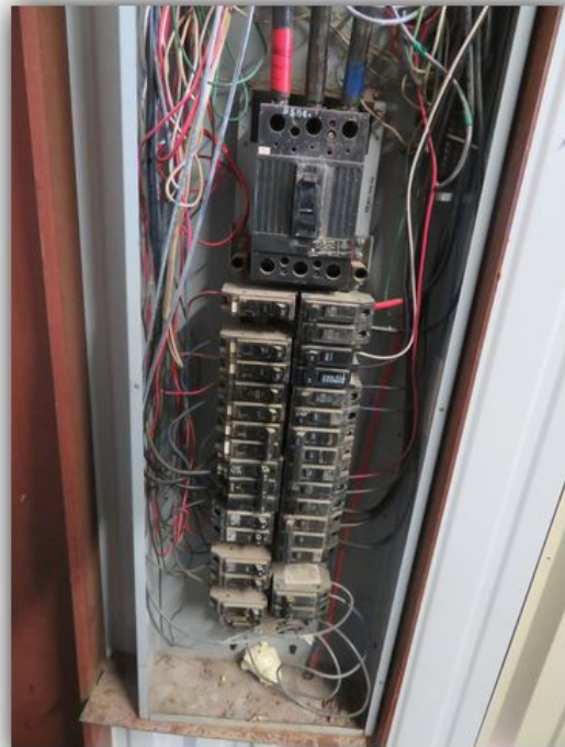
Far left panel has knock outs that need to be sealed and missing knock out strips on the inner panel.
