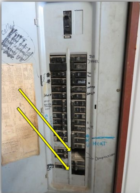
Seal the knock outs at the top of the panel. Safety issue
