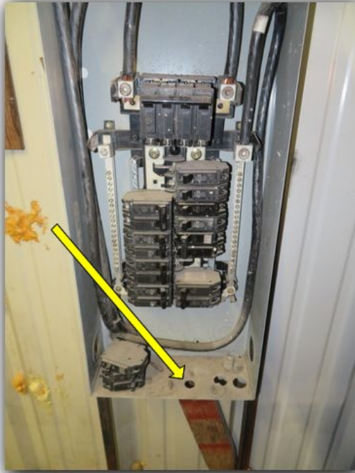
Far left panel has knock outs that need to be sealed and missing knock out strips on the inner panel.
