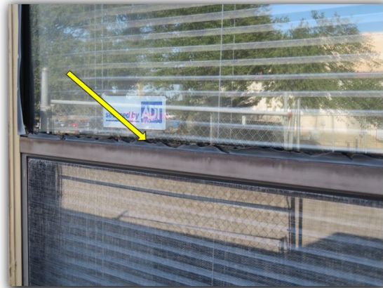
Right side office window has wood rot at the trim, thermal seal leak at the top window and the glazing strip beaten up.
