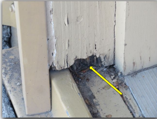
Right side office window has wood rot at the trim, thermal seal leak at the top window and the glazing strip beaten up.
