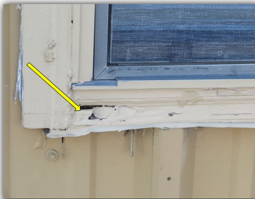
Right side office window has wood rot at the trim, thermal seal leak at the top window and the glazing strip beaten up.
